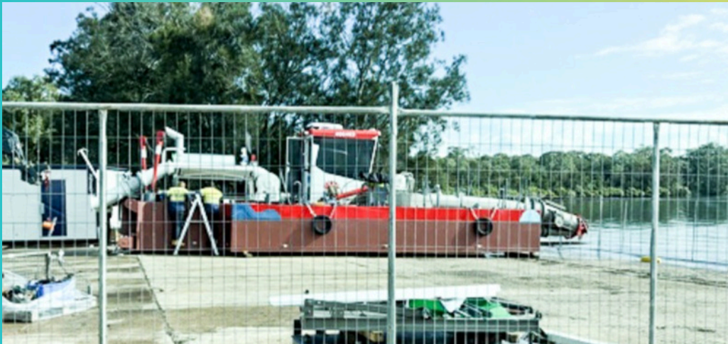
New dredge being assembled at Rathmines.
